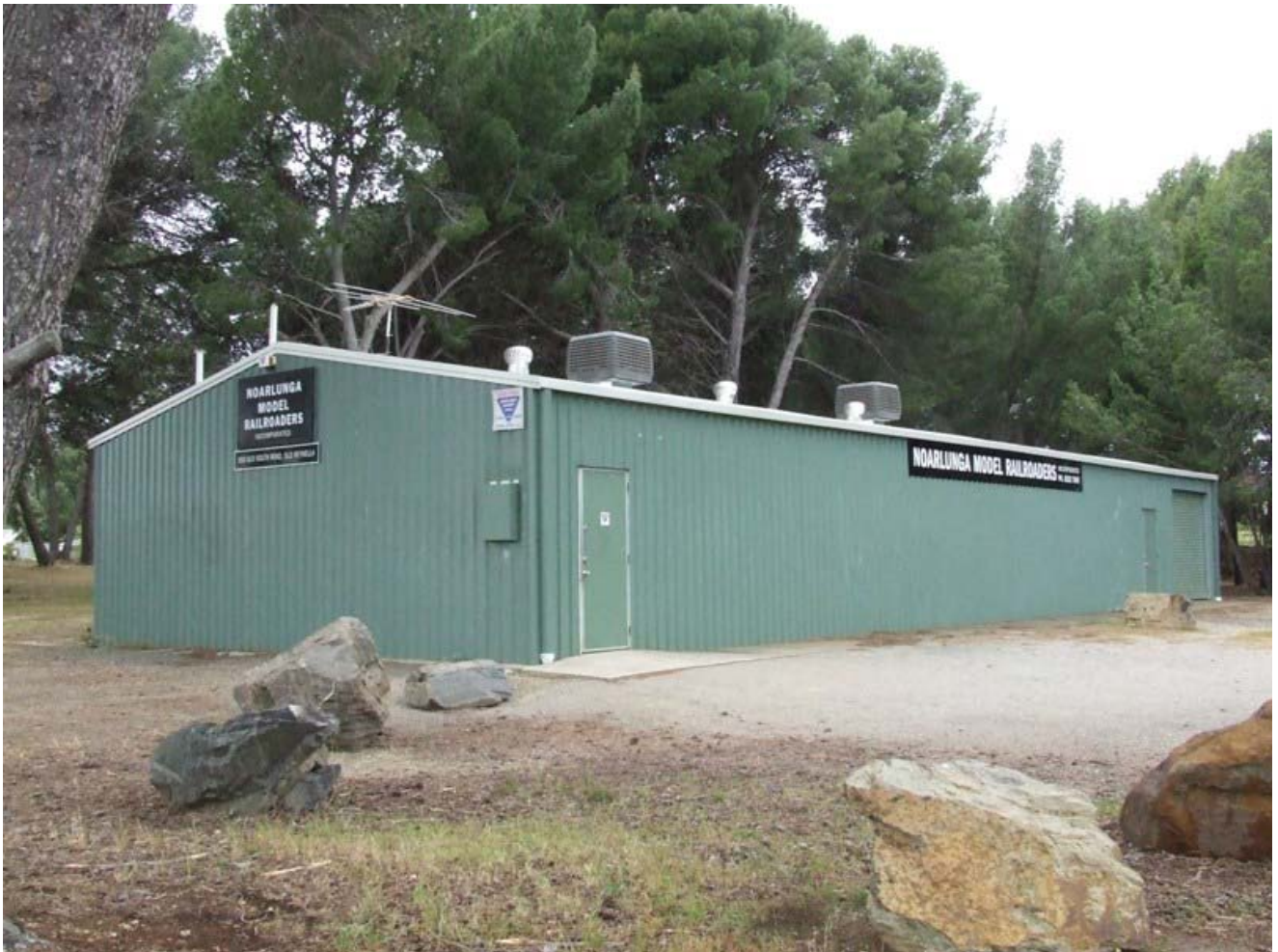
Above: Looks cooler already, our clubrooms soon after the installation of our new air-conditioners, I am almost wishing for some hot weather.
